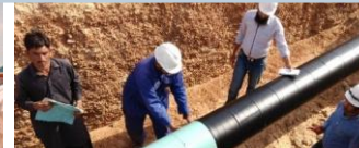
Pipeline coating & repair
