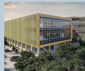
Inspiration Center in Brazil (Adhesive Technologies)
