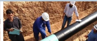
Pipeline coating & repair
