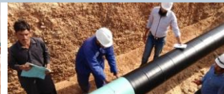
Pipeline coating & repair
