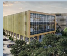
Inspiration Center in Brazil (Adhesive Technologies)
